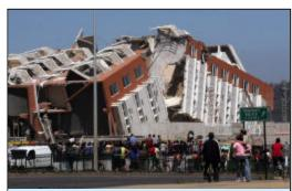
Gravitational collapse of a building leaves identifiable structures and chunks of material, not dust (Chilean earthquake Feb 28, 2010)
